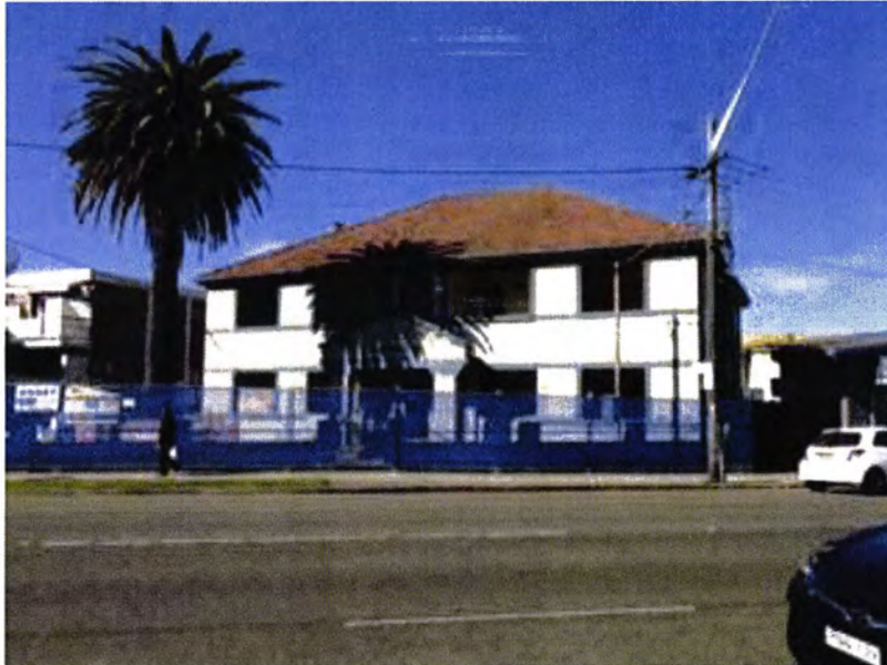
Figure 9: part of the site – 53 Forest Road, Hurstville
